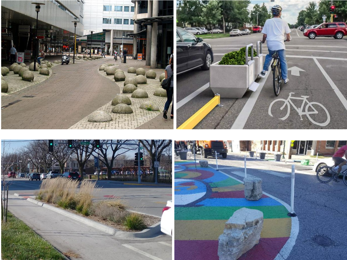
Figure 6: Representative photos of wide area bike protection options. Top left : Concrete spheres; Top Right : planter boxes; Bottom Left : curb island; Bottom Right : limestone blocks. (Picture Source: Street Smarts Design + Build, People for Bikes, WSP)
