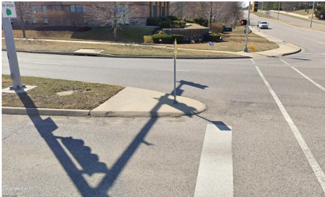
Figure 2: Example tapered median nose in Overland Park, KS (Image source: Google Earth)
