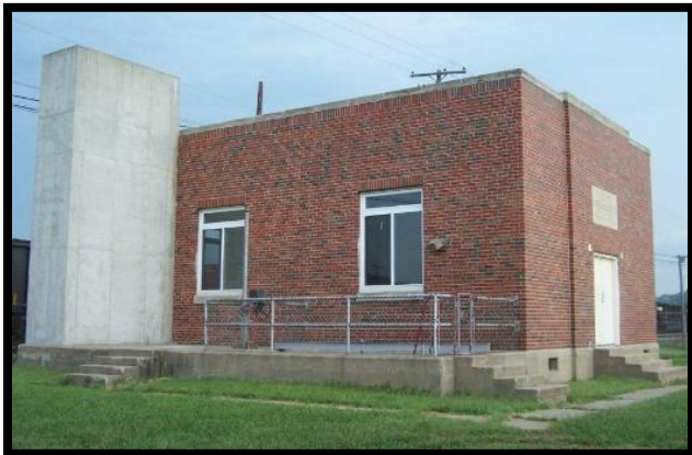
26 TH AVENUE PUMP STATION
