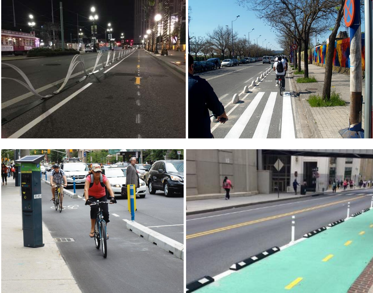
Figure 13: Representative photos of linear bike protection options. Top left: Wave Delineator, top right: bumps, bottom left: pre-cast curb, bottom right: wheel stops (Picture Source: Saris, People for Bikes, WSP)
