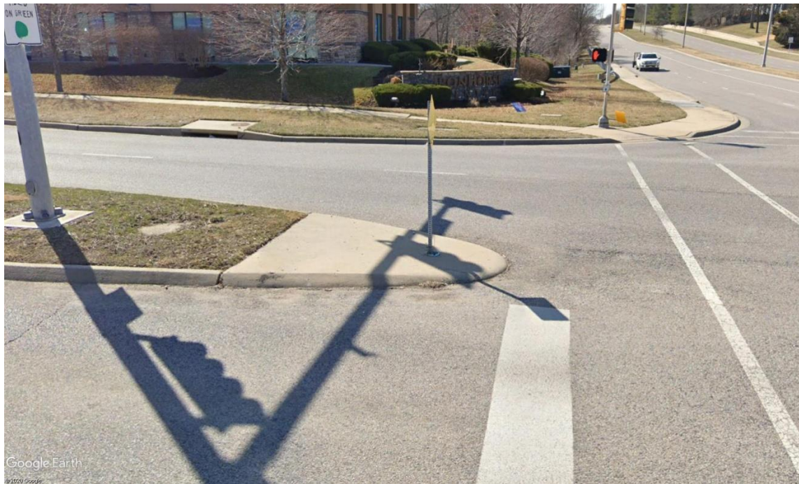
Figure 5: Example tapered median nose in Overland Park, KS (Image source: Google Earth)
