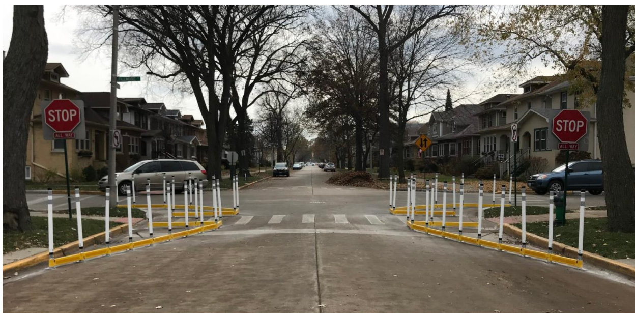
DeziLine's Curb Rail bump-out installation
