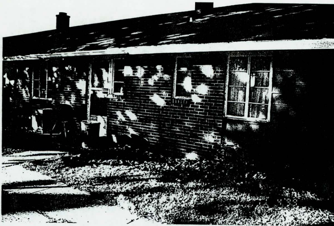
Rear Elevation of Building on 25th Avenue
