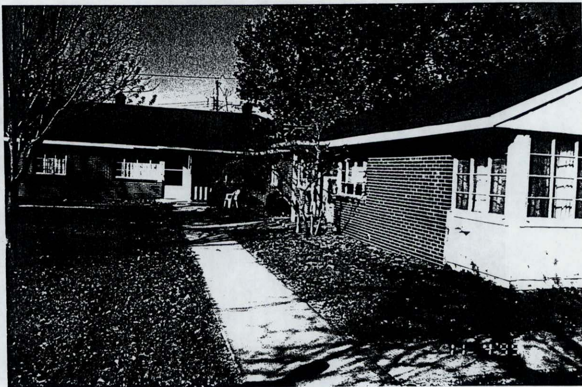
Front Elevation of Building on Swift
