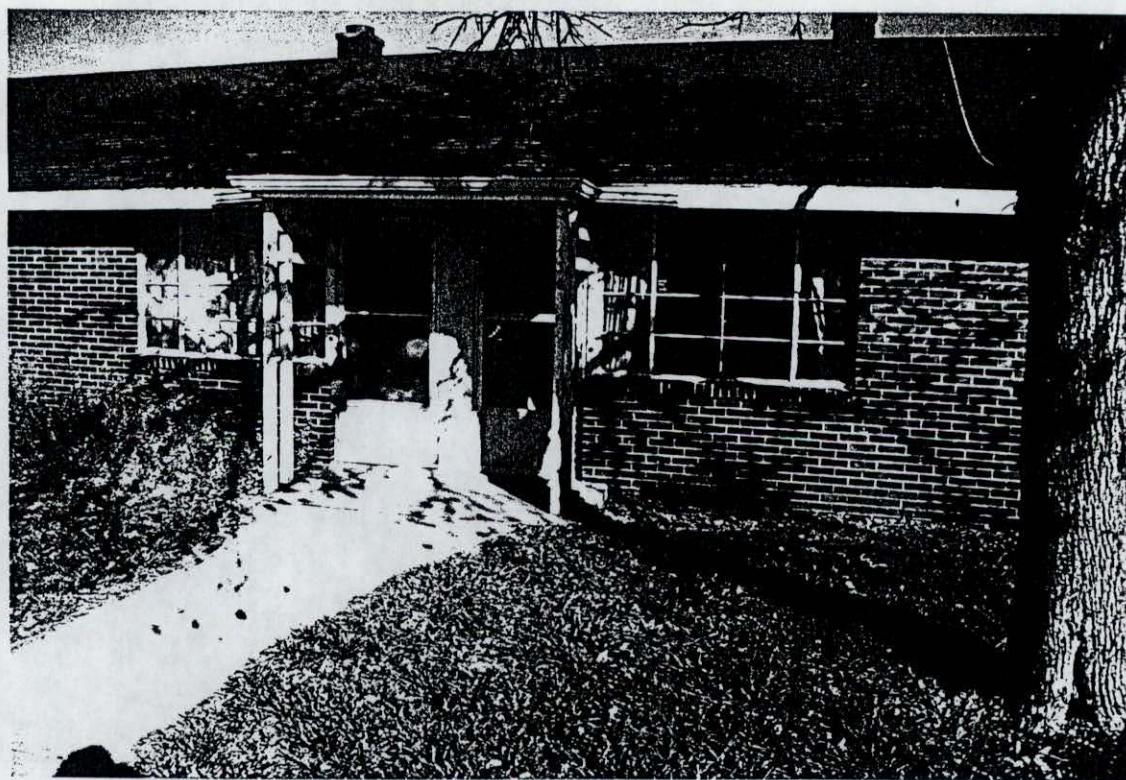
Front Elevation of Building on 31st Avenue
