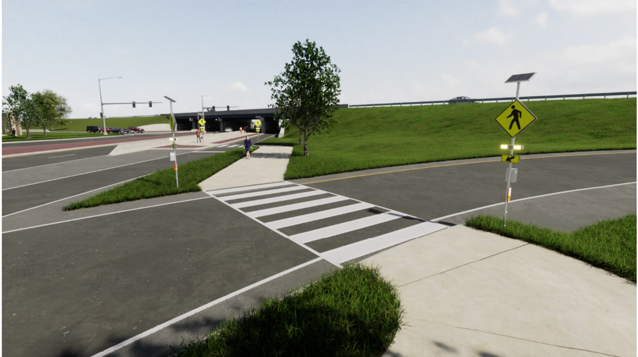
Figure 3: Rendering view of improved pedestrian crossing of ramp from eastbound Armour Road to southbound I-35 (looking east)
