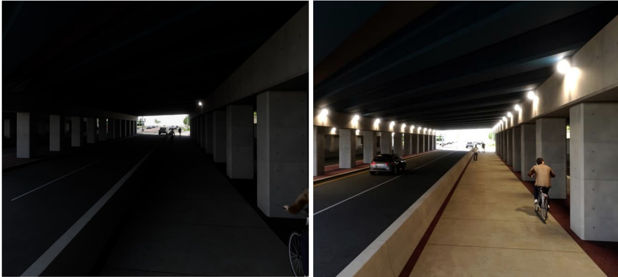
Figure 34: Rendering of how bridge appears in daytime with current lighting levels and tunnel standard lighting levels
