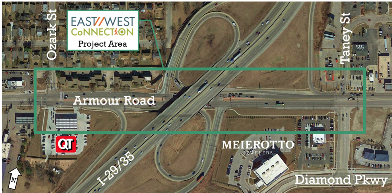
Figure 1: East/ /West Connection Study Area
