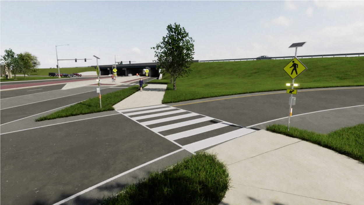
Figure 33; Rendering showing crosswalk of ramp from eastbound Armour to southbound I-35 with high visibility pavement marking, signs, and rapid rectangular flashing beacons
